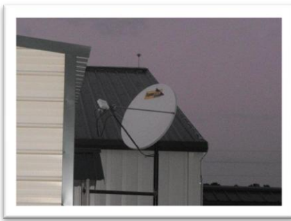
BC Antenna (Oil and Gas Operation)
